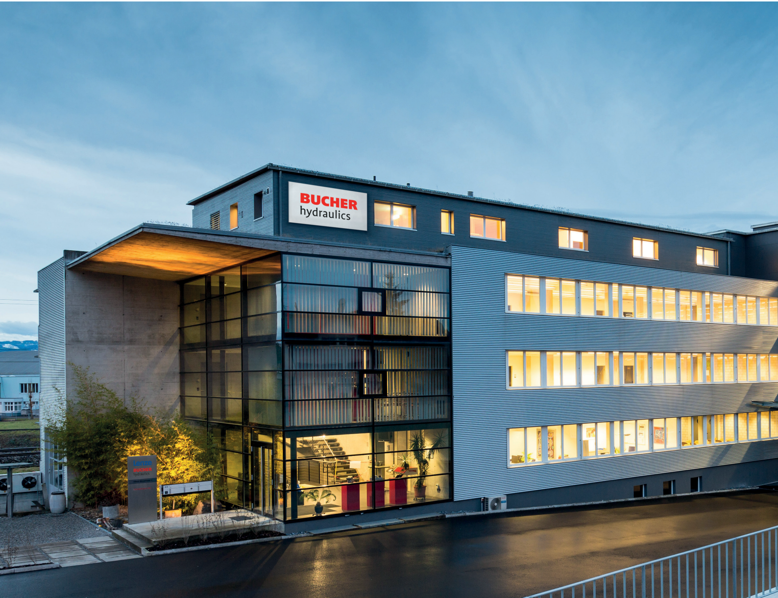
Bucher Hydraulics Mobile Drives in Romanshorn, Schweiz
